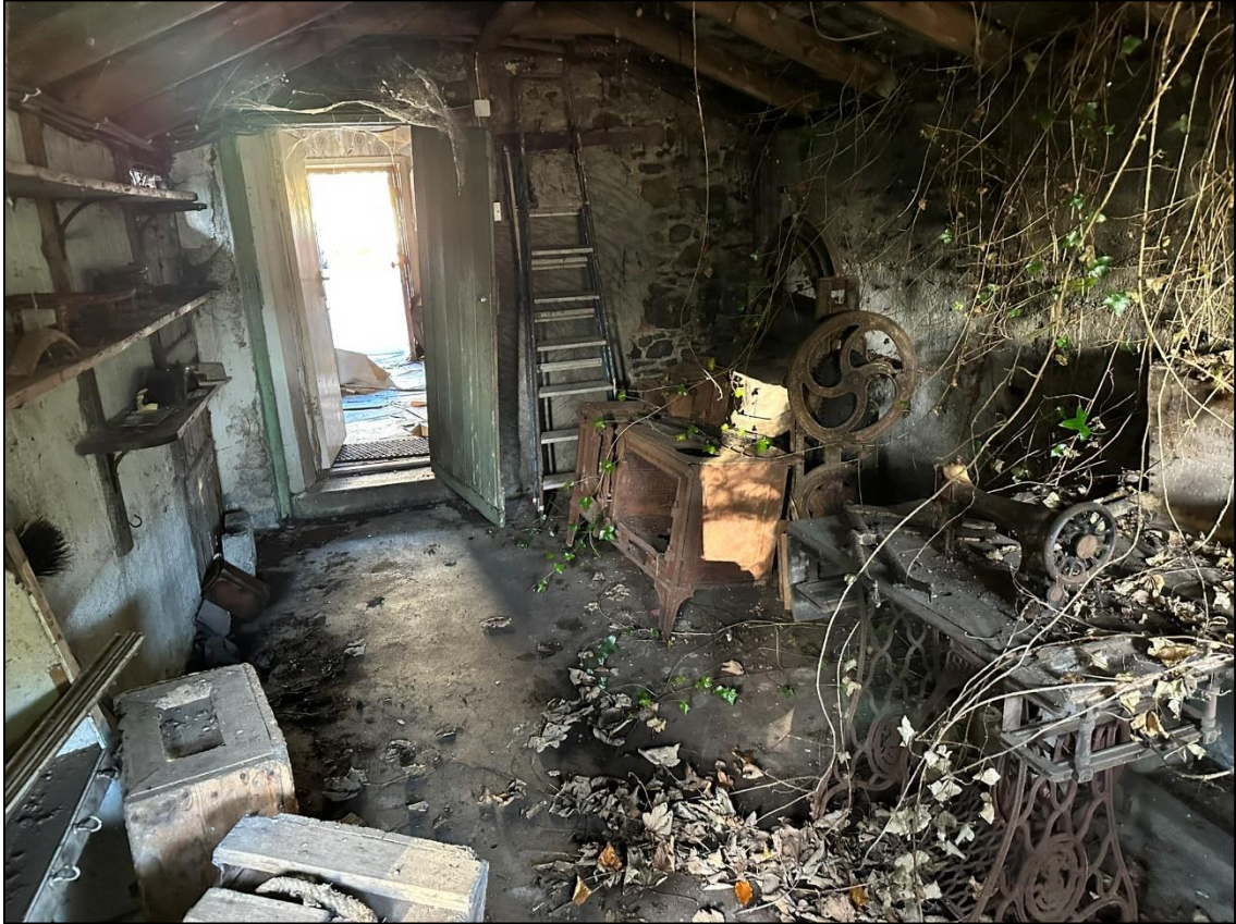
Plate 3 – Internal view of the derelict cottage (exposed to the elements)
